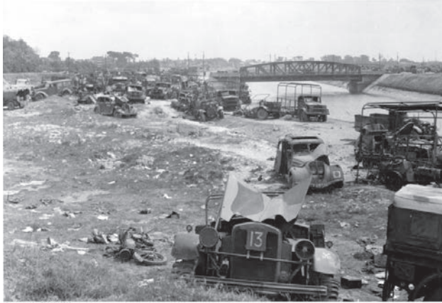
Figure 3. Destroyed equipment near Dunkerque ©Bundesarchiv
